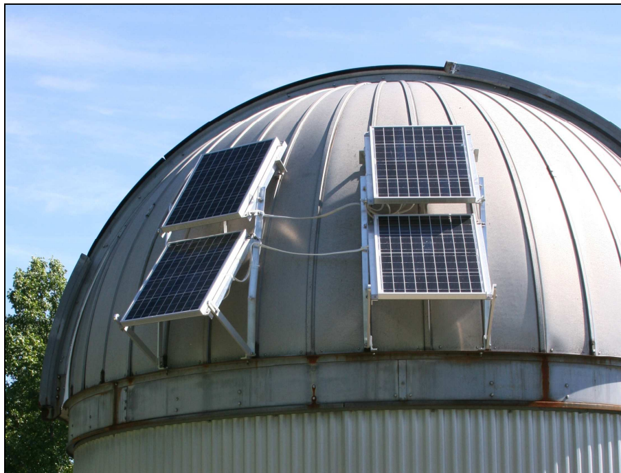
FIG. 33. The Kyocera solar panels mounted on the outside of the DSO-14 dome. (Author)
